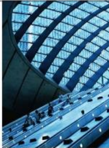
Figure 1: Escalators at Canary Wharf Station
