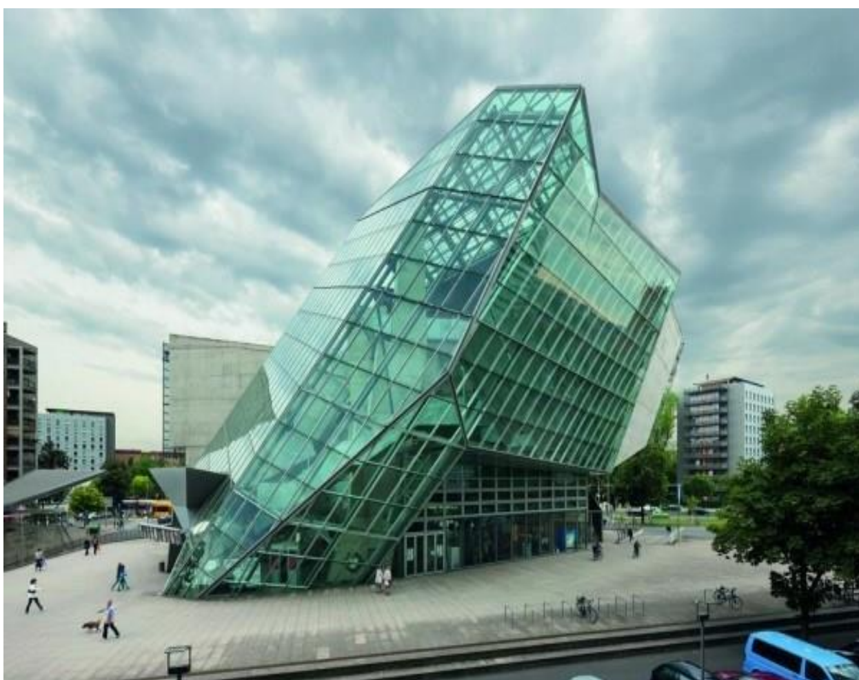
Architects: COOP HIMMELB(L)AU Project: UFA Cinema Center Location: Dresden, Germany Photography: Duccio Malagamba, Gerald Zugmann and H el ene Binet Client: UFA – Theater AG, D usseldorf, Germany
